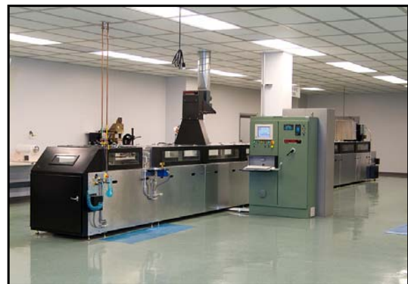
PROCAST Clean Room Installation
